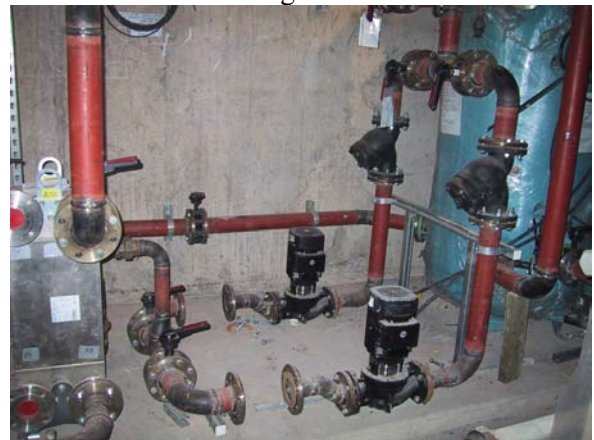
Partly installed heat exchanger and sink
