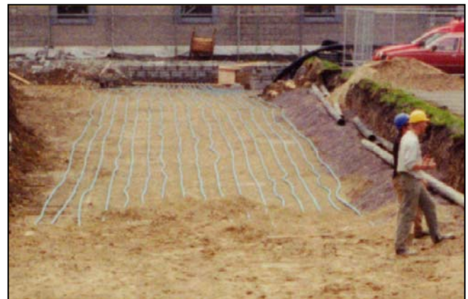
Horizontal Collector installation. (Courtesy Dunstar Ltd.)
