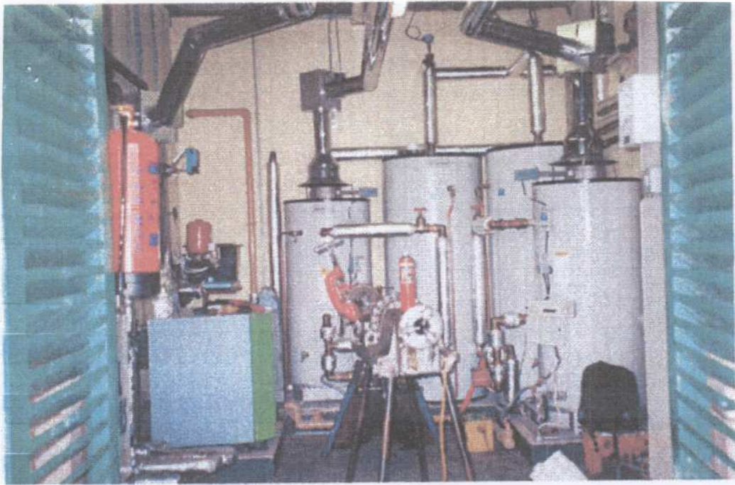
Boiler House at Sports Complex
